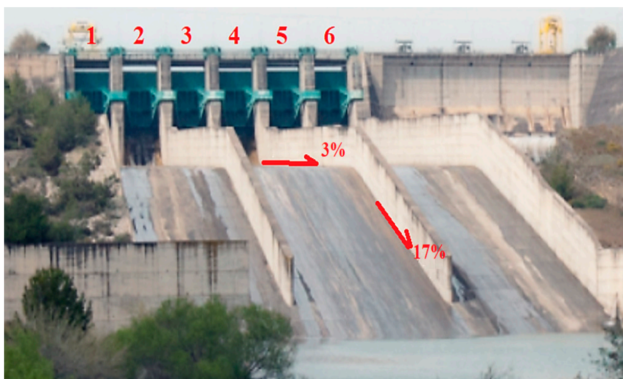
Figure 1. Çatalan Dam spillway structure. 1–6 numbers indicate chambers and arrows indicate 3% and 17% slopes in the discharge channel.
